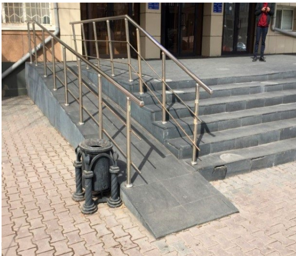
Figure 2. | A ramp designed to lift PWDs into institutions
